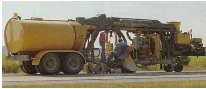
Figure 6. Large pavement grinding machine (from http://www.boartlongyear.com )
