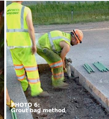
PHOTO 5: Grout bag method - pre-packed grout capsule & epoxy
