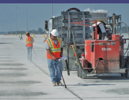
Crews working on a hot-pour sealant installation into 1/2-inch-wide longitudinal concrete pavement joints in a new intermodal facility in Joliet, Ill.
