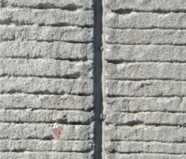
Joint sealants prevent water and incompressibles from entering into a pavement structure. Photos: Crafcro
