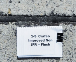
Low-modulus hot-pour sealant, located on a runway at Fairchild Airforce Base, in Washington state, is approximately 21 years old.
