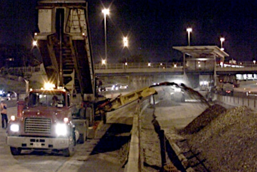
Conveyor shooting ballast during project
