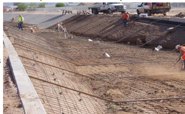
Application of FRC in a canal lining project significantly reduces labor requirements in the construction phase since the rebar or mesh layout phase is eliminated. Instead of using a longitudinal & transverse rebar layout or a welded wire mesh, FRC mix can be specified to meet system requirements at a much lower cost.
