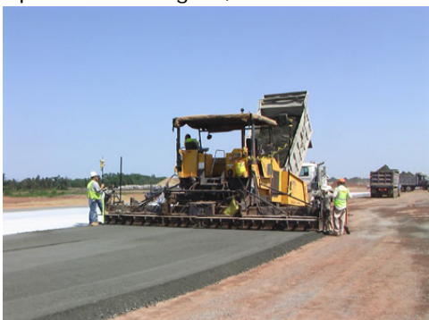
Placing CTB with high-density paver
