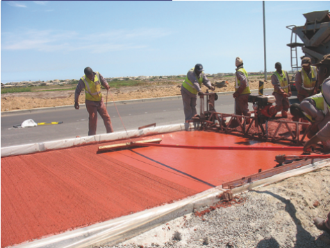
BRT bus lane constructed with a red-pigmented CRCP.
