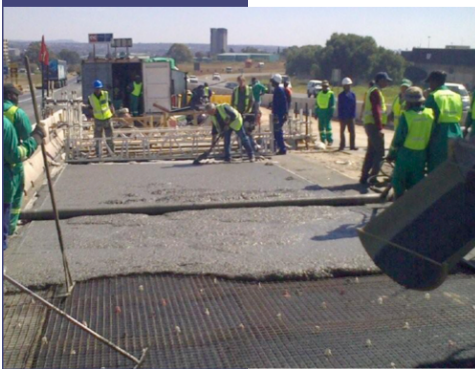
Placement of the Ultra Thin CRCP on the N12 national road in South Africa.
