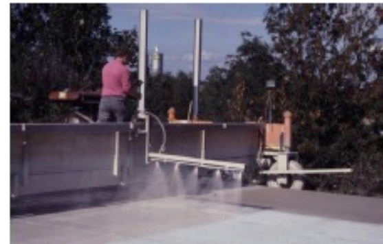
PHOTO: Applying surface retarder and curing compound
