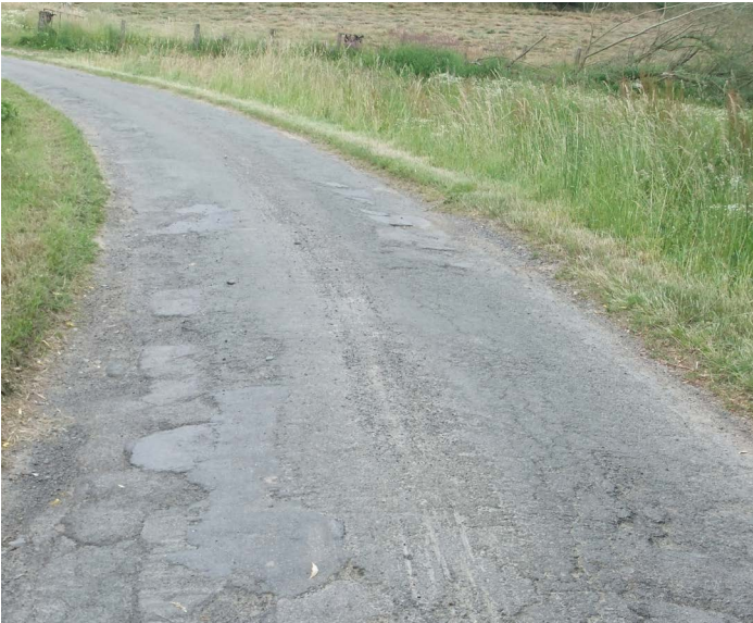
Deteriorated road surface.
