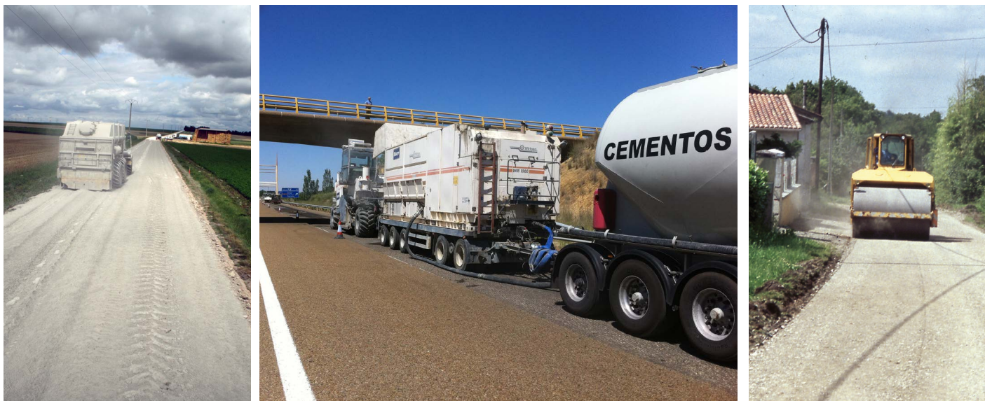
From left to right: spreading of a hydraulic binder – View of a recycling machine with cement slurry distribution – Compaction of the layer with a vibratory roller.
