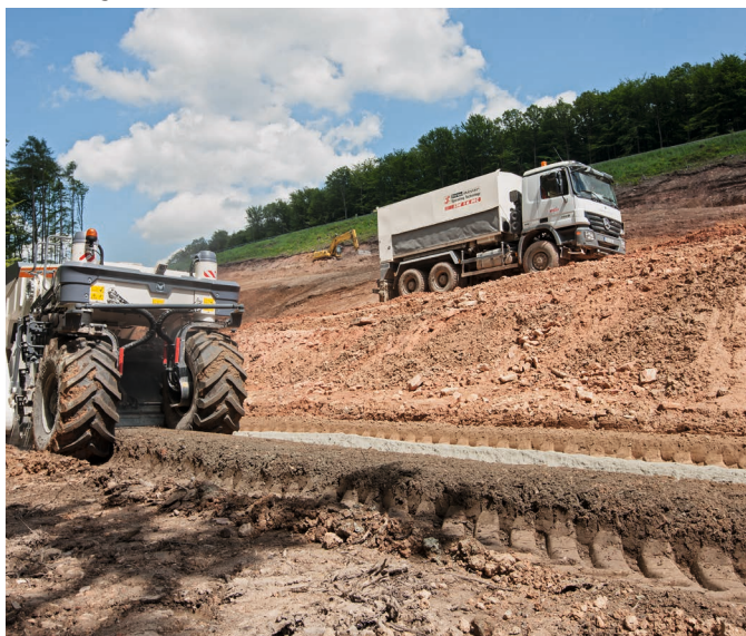
Soil stabilisation worksite.
