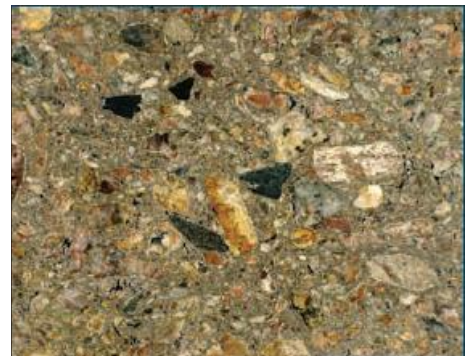
Figure 3: Roller Compacted Concrete (RCC)
