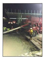
In fixed-form placements concrete is poured in areas where form boards have been placed in fixed locations around the perimeter of the slab, or pavement. Since concrete mixes are typically in a liquid state coming out of the mixer, these fixed forms contain the mix and provide shape until the concrete has cured enough to stand alone. In the picture to the left form boards have been removed
