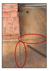
**SUGGESTION:** Risk of uncontrolled, random cracking can be reduced with preparation of a jointing plan as part of your concrete pavement design. We are available to help plan a joint layout for any project involving concrete pavement.
