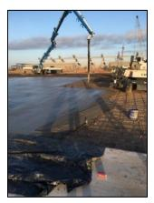
The use of concrete pumps, as shown in the picture to the left, is an effective way to extend the reach for discharge from a transit mixer, adding several feet of
