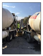
When mixers are used to deliver material for slip-form paving, the concrete is often discharged on the ground in front of the paver directly or by means of a conveyor similar to the picture to the left.
