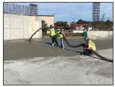
its compressive strength, and estimated California Bearing Ratio (CBR). By comparison, soils in the local area (Metro Atlanta and North Georgia) typically have CBR values ranging from 3 - 5, so an LDCC material at the lower end of the density range, can significantly improve support characteristics.
