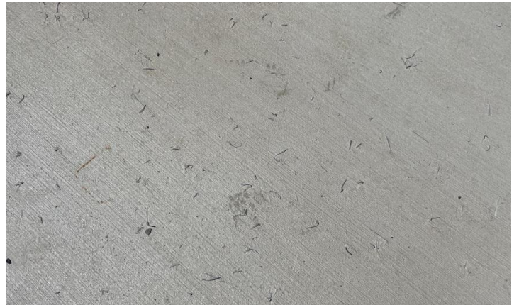
Figure 4: Close up of weakened shotcrete with dislodged macro synthetic fibres
