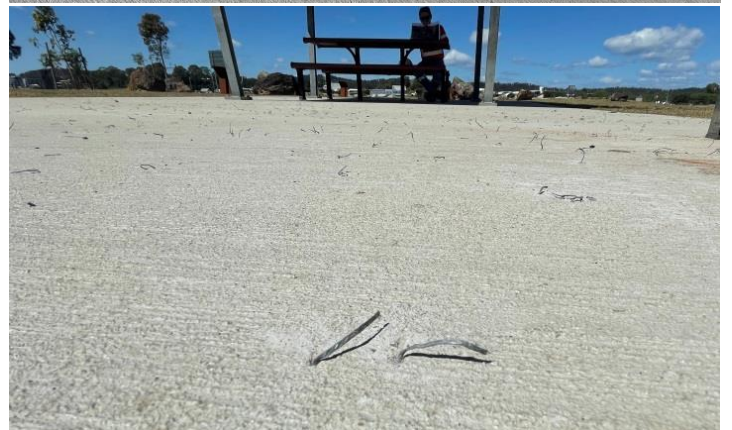
Figure 1: Concrete slab with protruding macro synthetic fibres.
