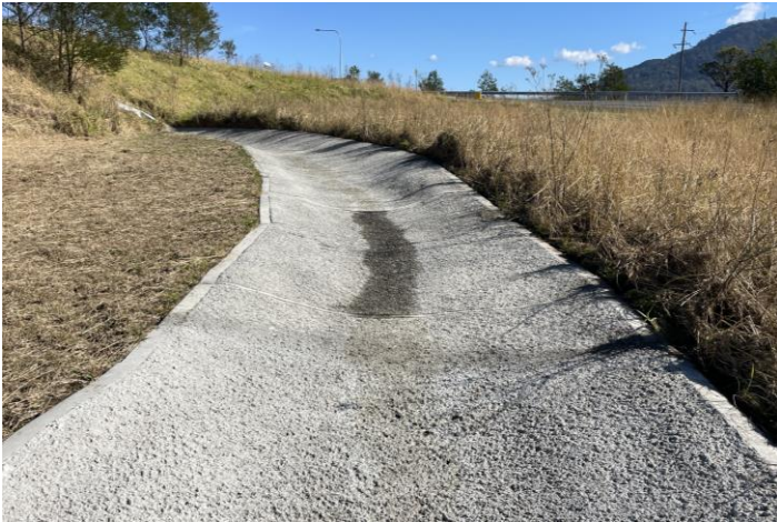
Figure 2: Shotcrete with macro synthetic fibre reinforcement, shortly after application.
